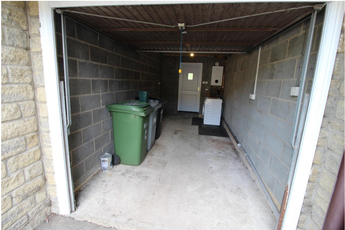
Garage with access to the rear garden plus gas boiler and washing machine.
